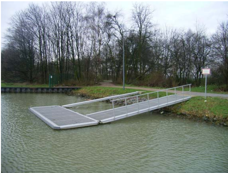
Pontoon with land access
