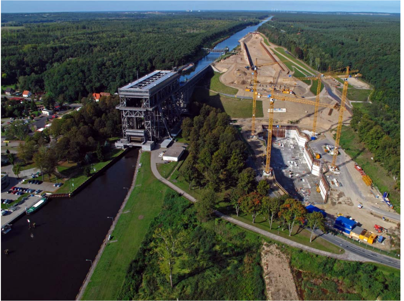
Figure 14. Construction site in August 2010
