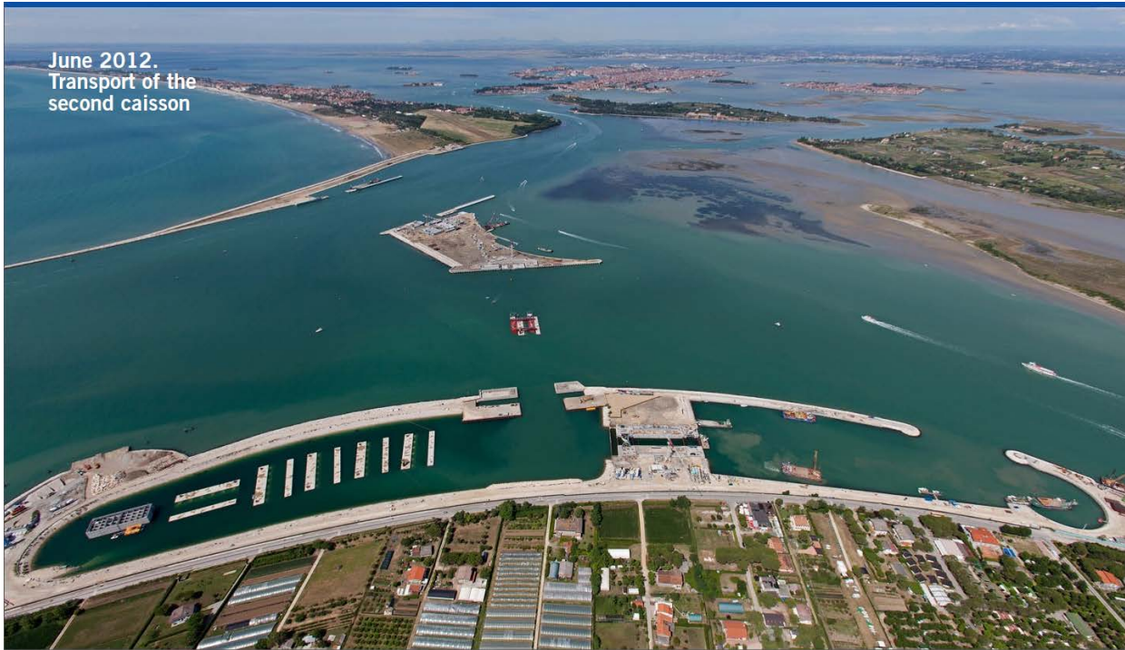
Fig.4 Installation of foundation caissons at Northern lido inlet, June 2012.
