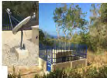
Unmanned stations with satellite communication
