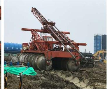
In-situ treatment of dredged materials for Port of Valencia, Spain. A working platform was formed on top of muddy deposit ( $c_u=75$  kPa)
