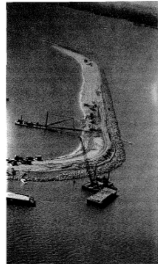
Fig. 5.3 : Construction of the Hart-Miller Island disposal area in the U.S.A. The dike was protected with layers of rock of increasing sizes. (With kind permission of Great Lakes Dredge & Dock Company).
